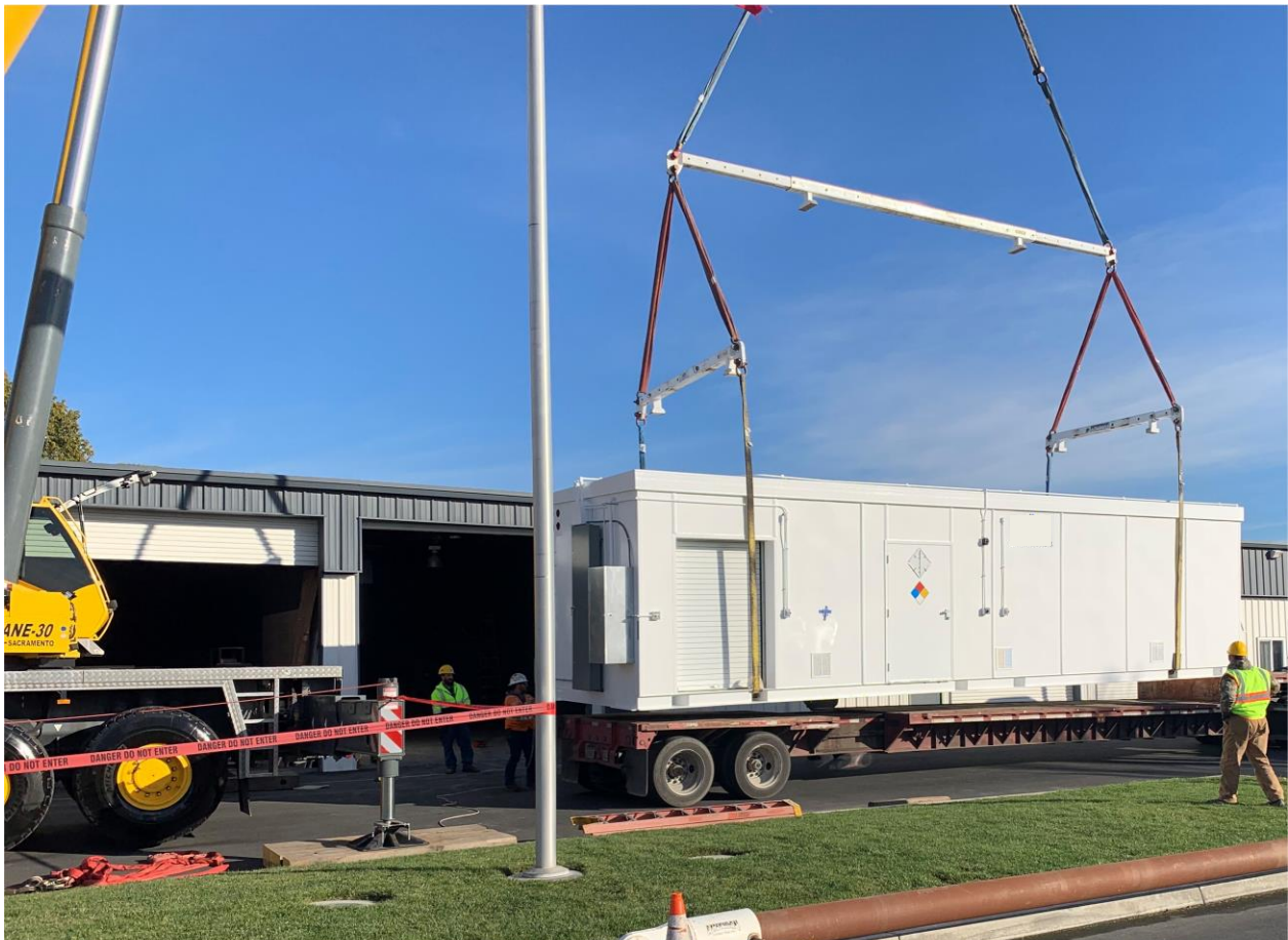
Extraction Equipment being lifted off truck in Ceres, CA
